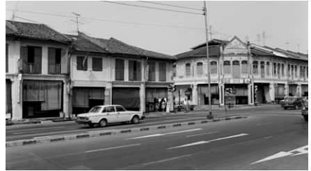
Shophouses along Balestier Road at the Kim Keat Road junction, 1982 From the Lee Kip Lin Collection. All rights reserved. Lee Kip Lin and National Library Board, Singapore 2009.
