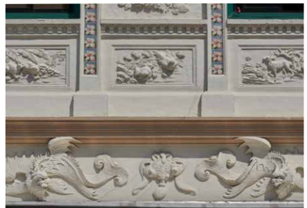
Close-up of motifs on the Kwan Yow Luen shophouses, 2018
